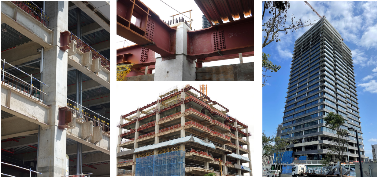
Figure 8: A 27-storey New RCS building in Nangang, Taipei by Ruentex Engineering and Construction Co., Ltd.
